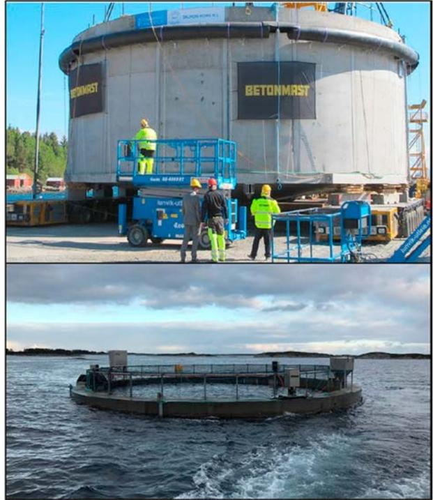
Figure 58: Concrete containment fish tank (Picture courtesy of Tor Ole Olsen).
