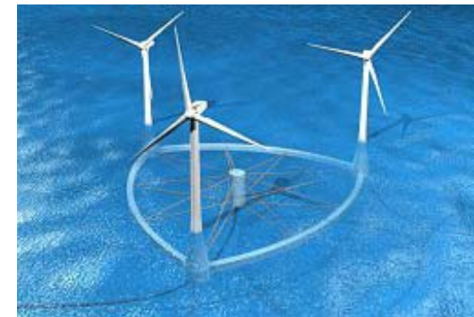
Figure 2.4.2: Semi-sub Type Floating Wind Turbine (Phuc & Ishihara, 2009)
