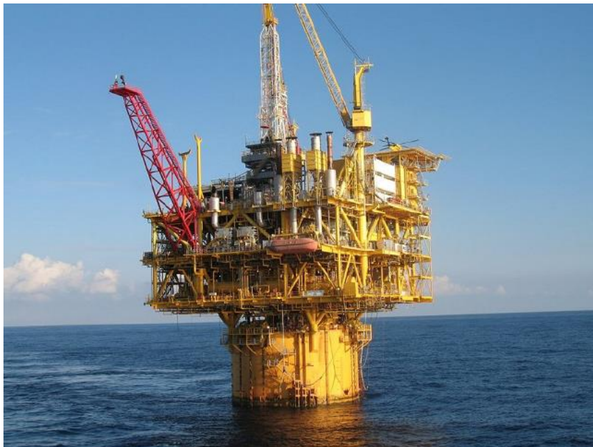
Figure 9-11: Spar Platform.
