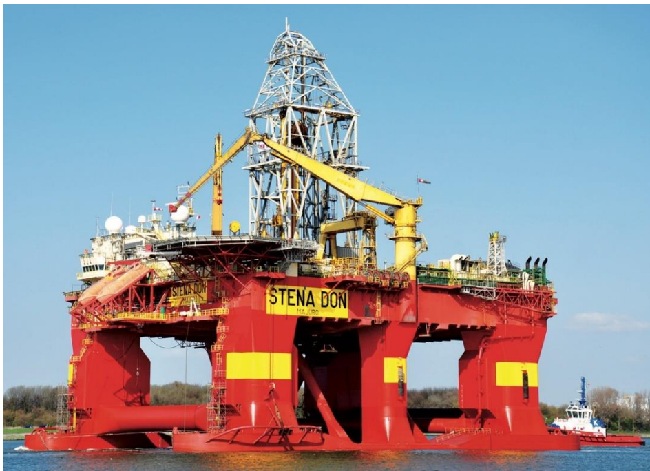
Figure 9-3: Semisubmersible Drilling Unit.
