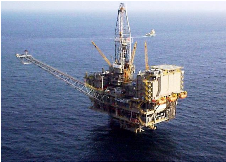
Figure 9-9: Flexible Platform/Compliant Tower.
