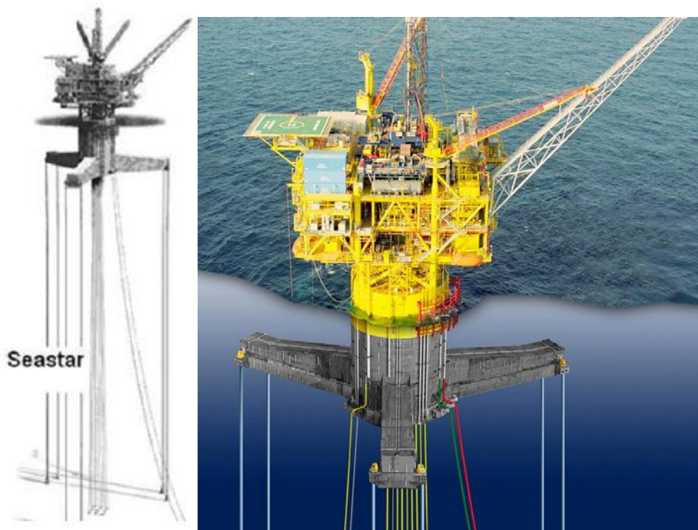
Figure 9-12: Tension Leg Platforms.
