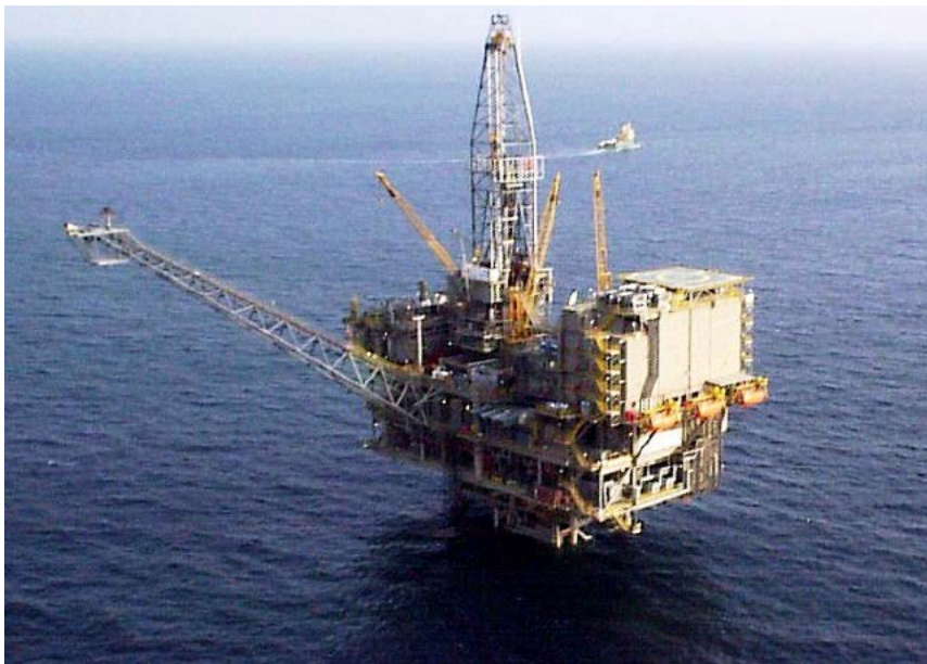
Figure 9-9: Flexible Platform/Compliant Tower
